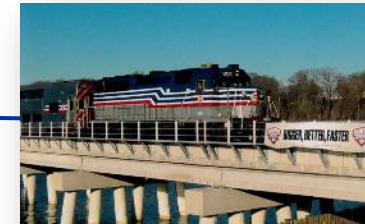
Quantico Bridge Opens (2007)
