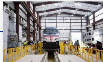
LOU Facility Opens (2023)
