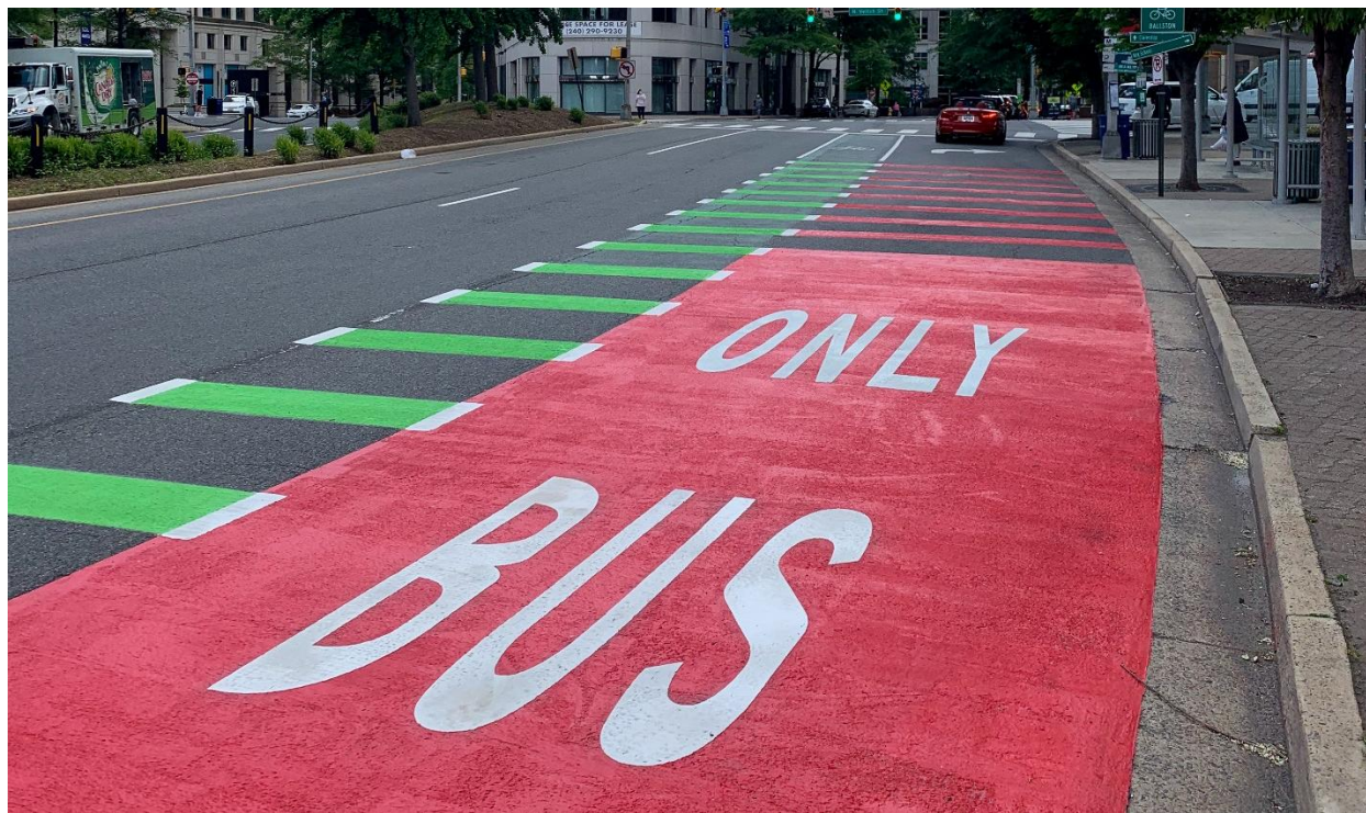
Figure 10: A location in the Court House area of Arlington that has adjacent bus and bike lanes
