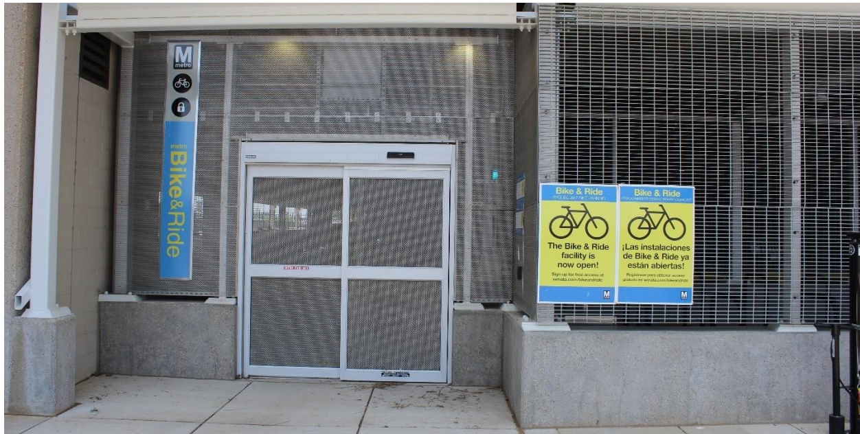
Figure 2: Secure bicycle parking at a Metro station
