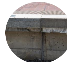
West Falls Church Platform Before Improvements
