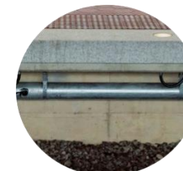
West Falls Church Platform After Improvements
