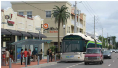
Downtown bus stop with off-board fare collection, shelter, and real-time information
