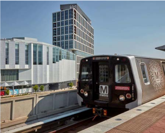
McLean Metro Rail Station, Fairfax County
