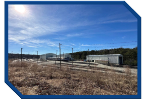
Crossroads Yard Future Phases ($48 million)
