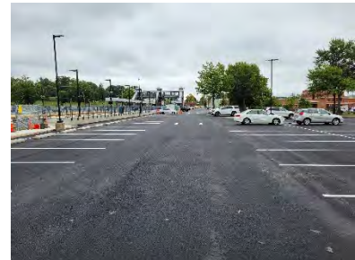
Quantico station parking lot paving and striping
