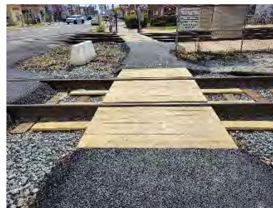
Temporary timber pedestrian crossing at the Quantico station.
