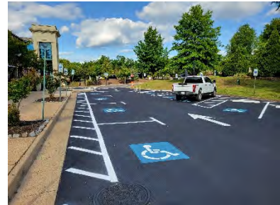
Sealcoating & restriping at Fredericksburg
