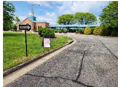
Proposed pavement sealcoating and restriping at Woodbridge.
