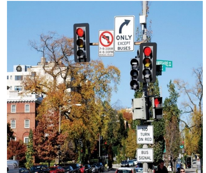
A Bus Priority Queue Jump Signal in DC
