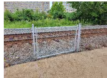
Chain link gate replacement at Alexandria station
