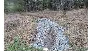
Placement of drainage stone
