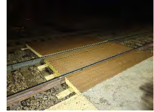
Replacement of timber crossing
