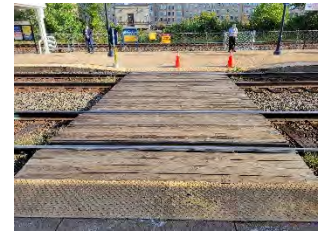
Crossing to be removed and reinstalled at Alexandria station
