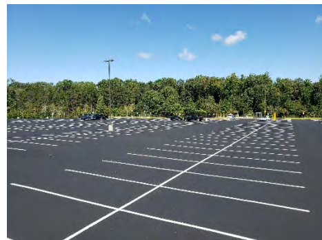
Leeland Road station pavement repairs and restriping (after)
