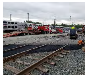
Grade-crossing paving at Crossroads as part of the LOU.
