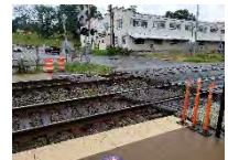
Repaired timber pedestrian crossing
