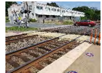
Fire-damaged timber pedestrian crossing
