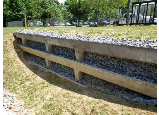
Repairs to Erosion Near Retaining Walls at Leeland Road Station (1)
