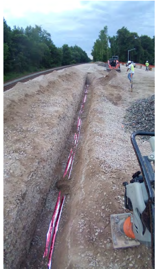
Electrical and communication conduits are installed in advance of construction of the platform extension at Lorton.
