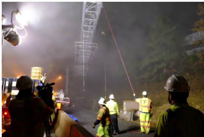
The first toll gantry on I-66 inside the Beltway is lifted into place between exits 71 and 72 in Arlington.
