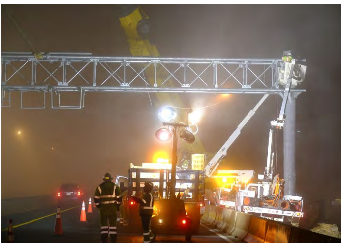
Crews install the first of eight toll gantries on I-66 inside the Beltway in the early morning hours of January 18, 2017.
