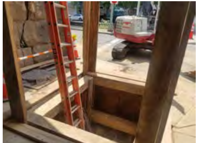
External trenches are being installed north of the VRE L'Enfant Station in order for the storage track to be equipped with electrical power, and ultimately make the track operational.
