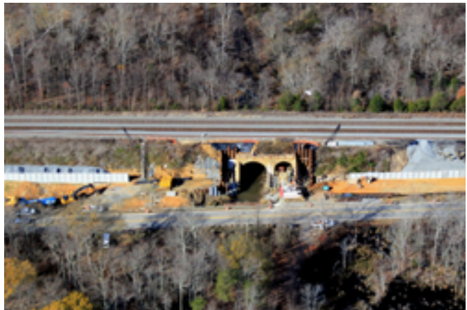
Preparations are made for laying the foundations for the new arch extensions spanning Massaponax Creek that will support the new third track.
