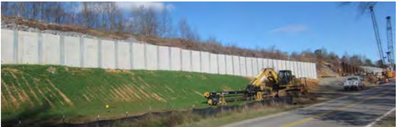
Retaining wall and embankment/trackbed construction progress north of Massaponax Creek.
