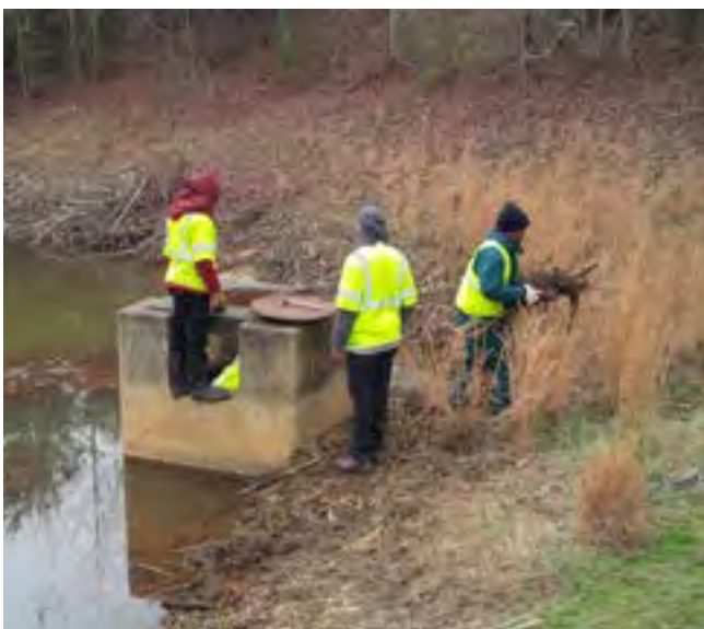
Removal of beaver-related debris at Crossroads Yard stormwater pond.
