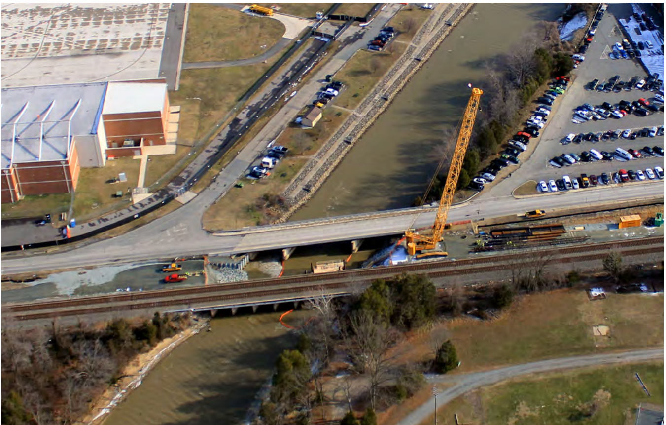
Work proceeding on a new bridge for the third track over Chopawamsic Creek.
