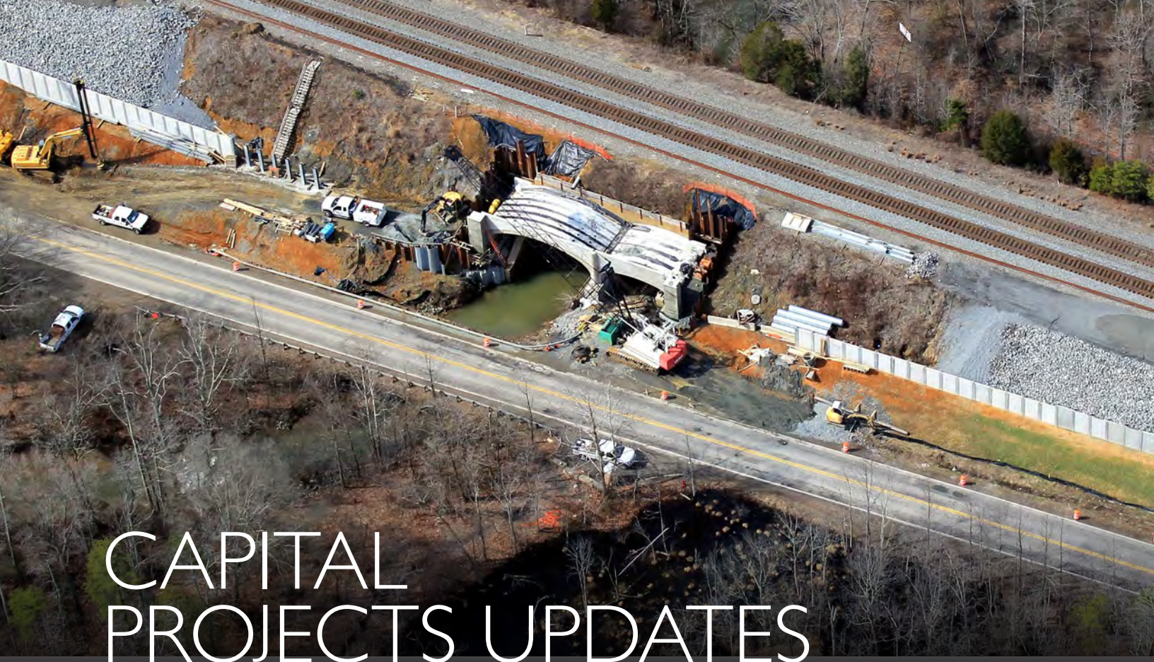
Progress on retaining walls, arch extension and trackbed at Massaponax Creek.
