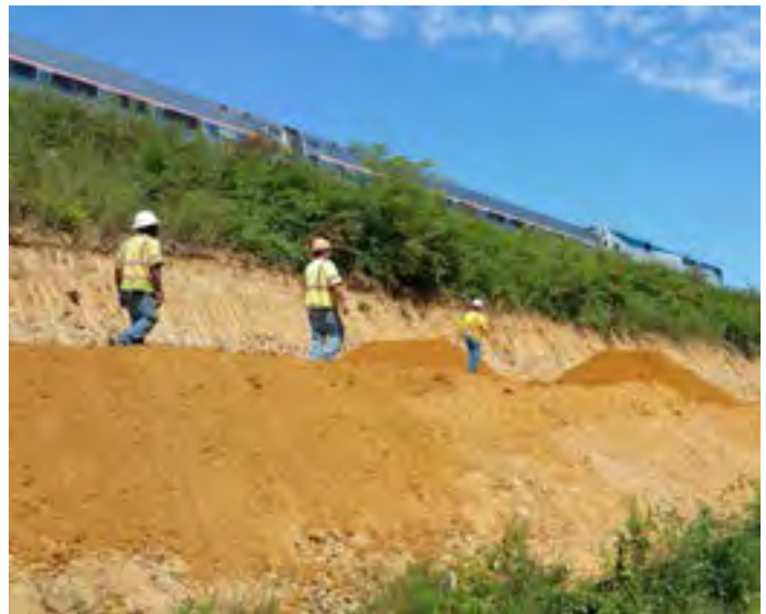
Just down the road, an Amtrak train rolls past VRE crews building up the subgrade for a new third track on the CSXT's RF&P Subdivision.
