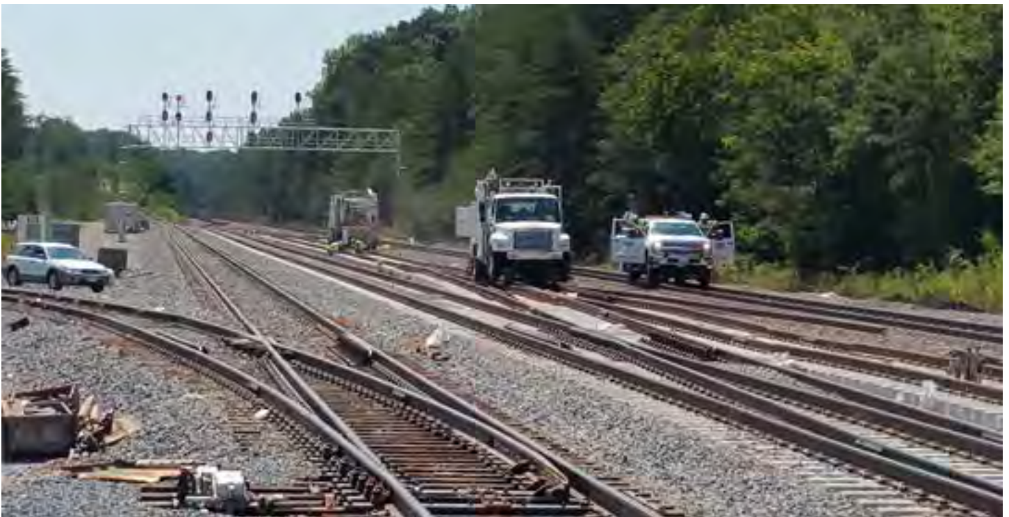
Further south, CSXT track and signal crews are modifying Crossroads Interlocking on the RF&P Subdivision in preparation for the Phase 2 cut-in of the new third track that VRE is constructing planned for the end of September.
