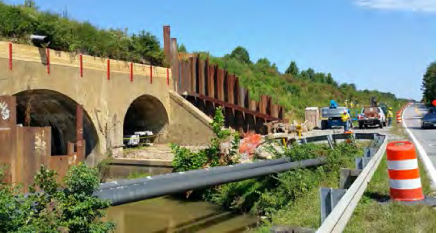
A short distance down Benchmark Road, VRE's contractor is back at work, extending the arches over Massaponax Creek to support a future third track on the CSXT RF&P Subdivision. Project completion is scheduled for the last quarter of 2015
