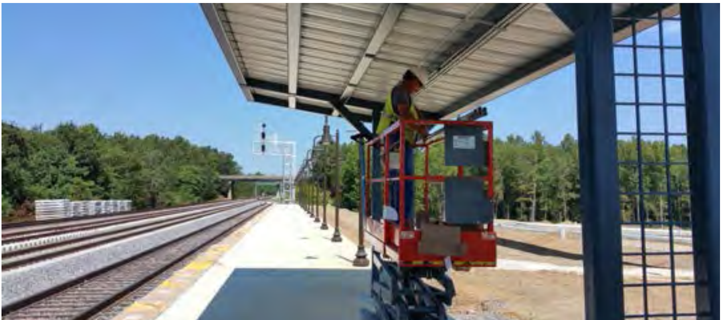
The Electrician from VRE's contractor CFS Service Corporation works atop a scissor lift to run wire conduits at the new VRE Spotsylvania Station. The new signal gantry at the north end of the platform controls access onto the CSXT Main Line from the spur track serving the station platform and VRE's Crossroad Maintenance and Storage Facility.
