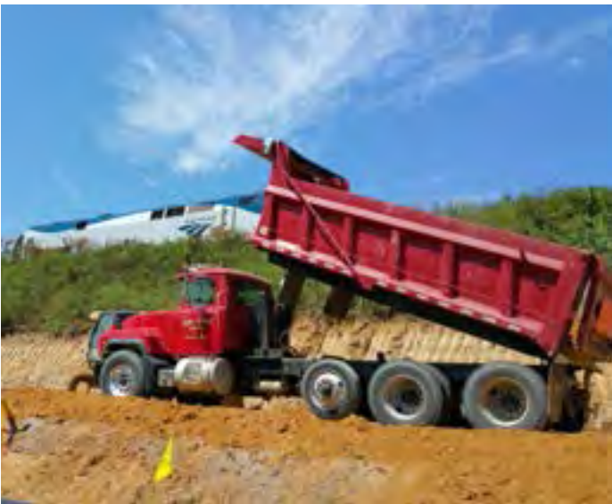
VRE's contractor delivers fill on the worksite for the subgrade to support a new third track for the CSXT RF&P Subdivision as an Amtrak train passes by.
