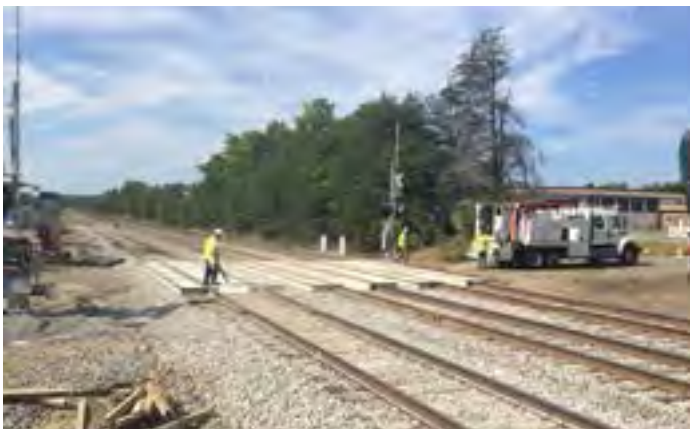
Precast roadway panels are bolted in place as the rehabilitated grade crossing at Mine Road nears completion.
