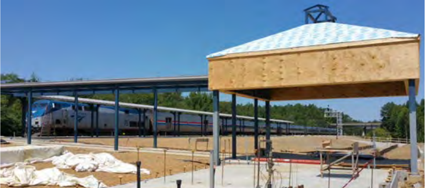
An Amtrak train passes the new VRE Spotsylvania Station as the station headway and platform canopy begin to takes shape. The concrete slab for the station waiting room is in the foreground.
