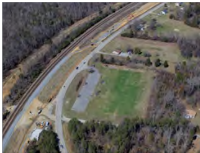
Track bed is graded and in place, awaiting installation of track along Benchmark Road in Spotsylvania County.
