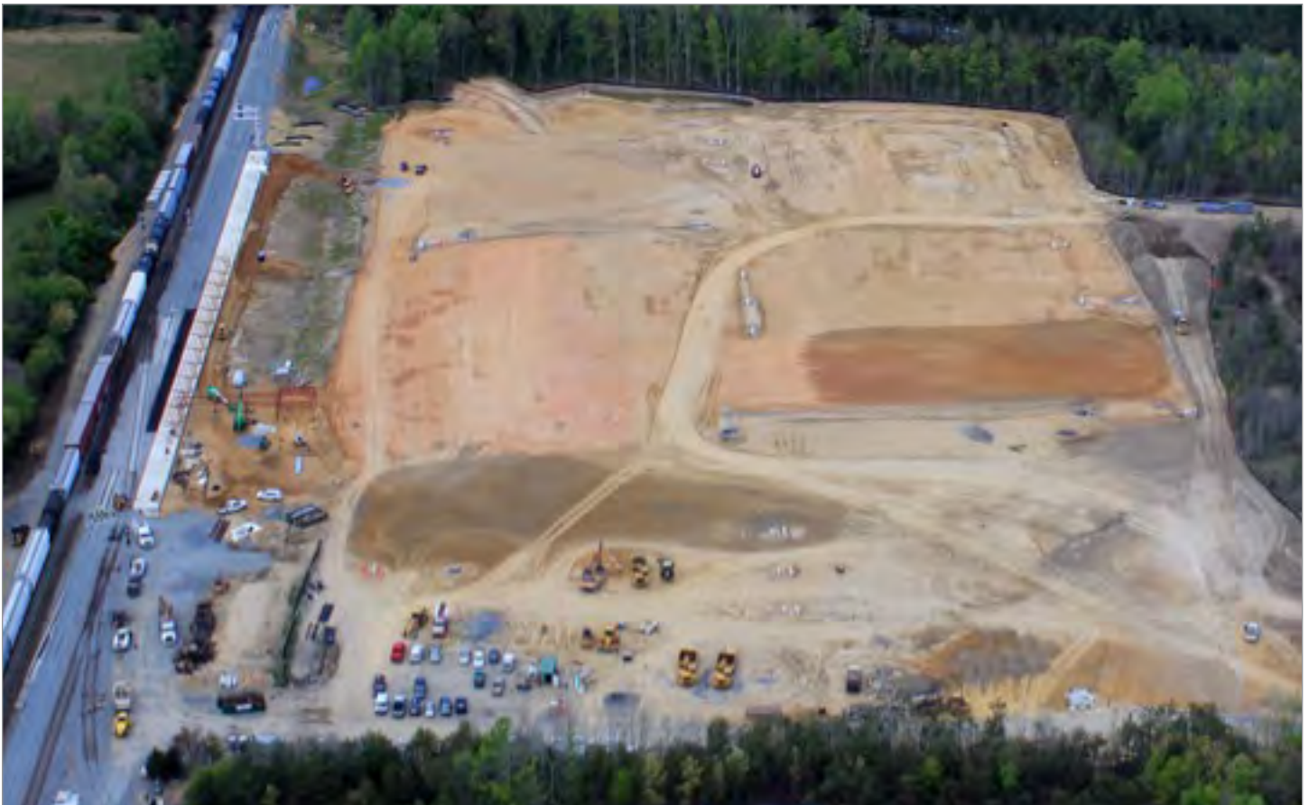
Adjacent to the new Spotsylvania Station platform on the left, the County's contractor is completing site grading and installing drainage in preparation of paving the 1,500-car parking lot.
