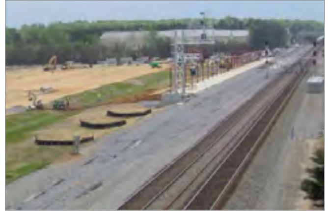
With concrete platform work complete, the new Spotsylvania Station begins to take form. From right-to-left, the picture shows the two active CSXT main line tracks and (peeking out from under stone ballast) the new third main line track, and the new platform track that also leads to the VRE Crossroads Maintenance and Storage Facility.
