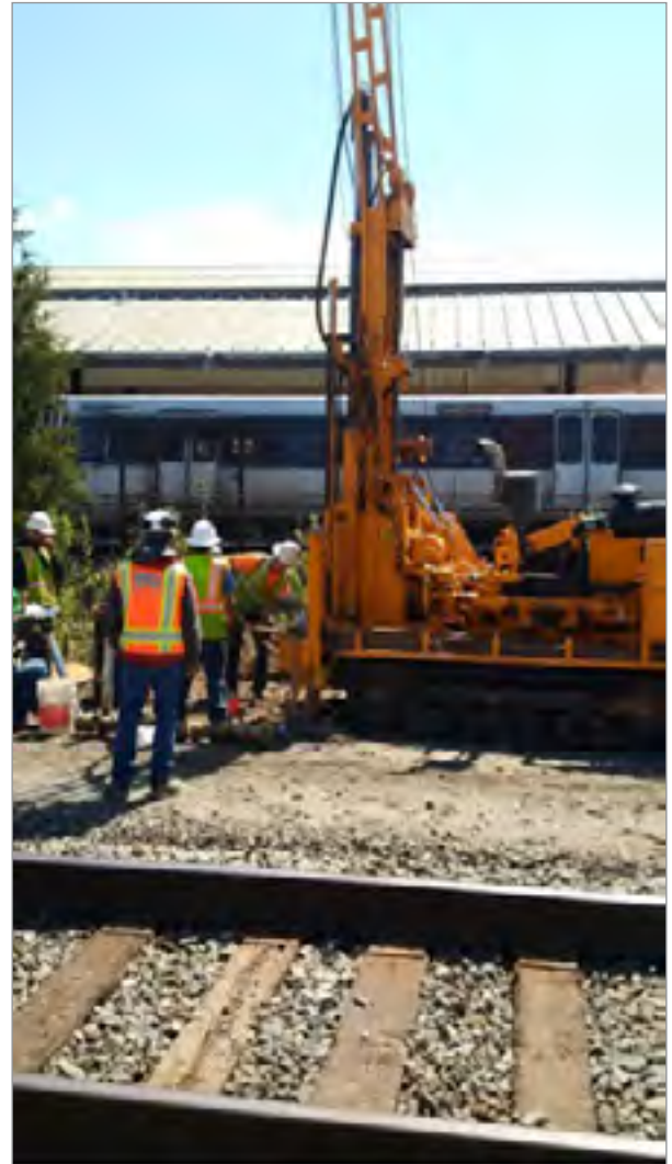
The VRE geotechnical contractor collects soil borings along the future tunnel alignments between at the Alexandria Union Station and the King Street Metrorail stations to determine subsurface conditions for engineering.
