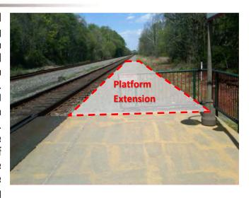
parking lot to the extended platform. The platform design is substantially complete and has been submitted to Fairfax County for permitting. Construction is expected to begin in summer 2013 and be complete in fall 2013.
