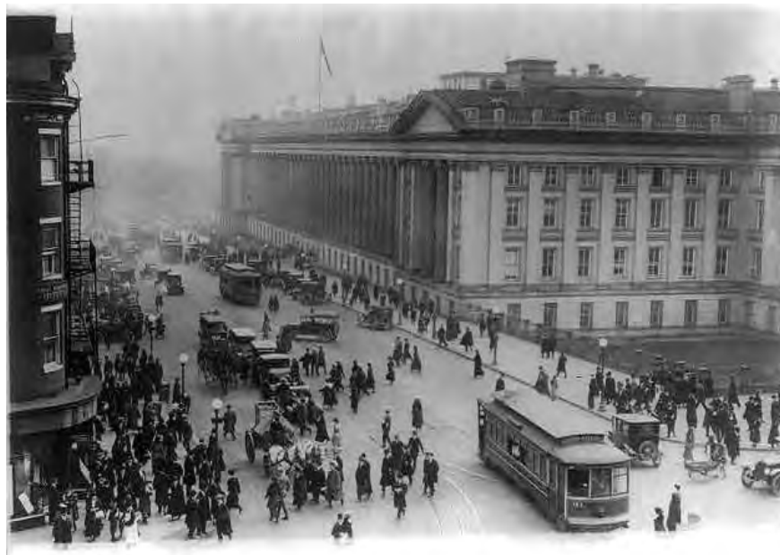
Streetcars ply Pennsylvania Avenue and 15th Street alongside the U.S. Treasury Building.
