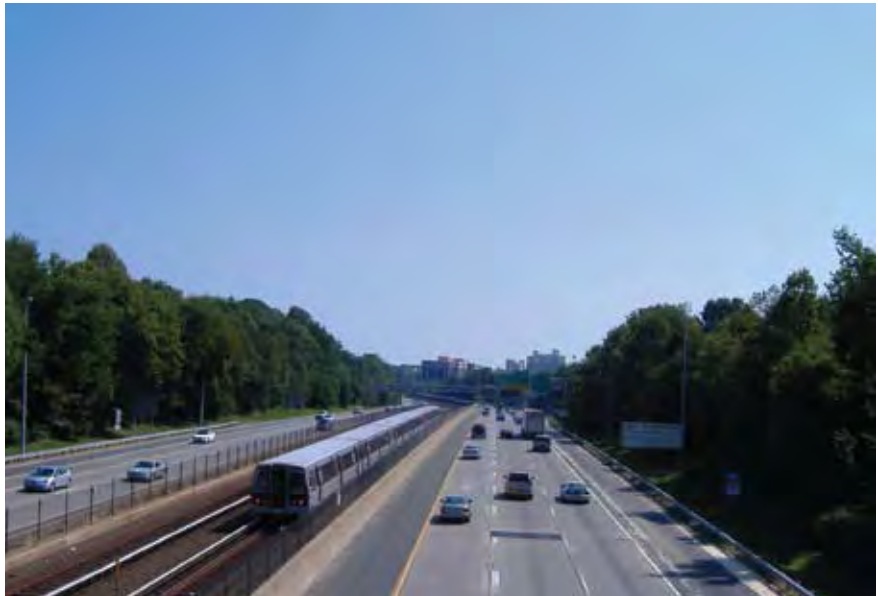
The system sits above ground in Virginia's Fairfax County alongside I-66, just outside the Beltway.
