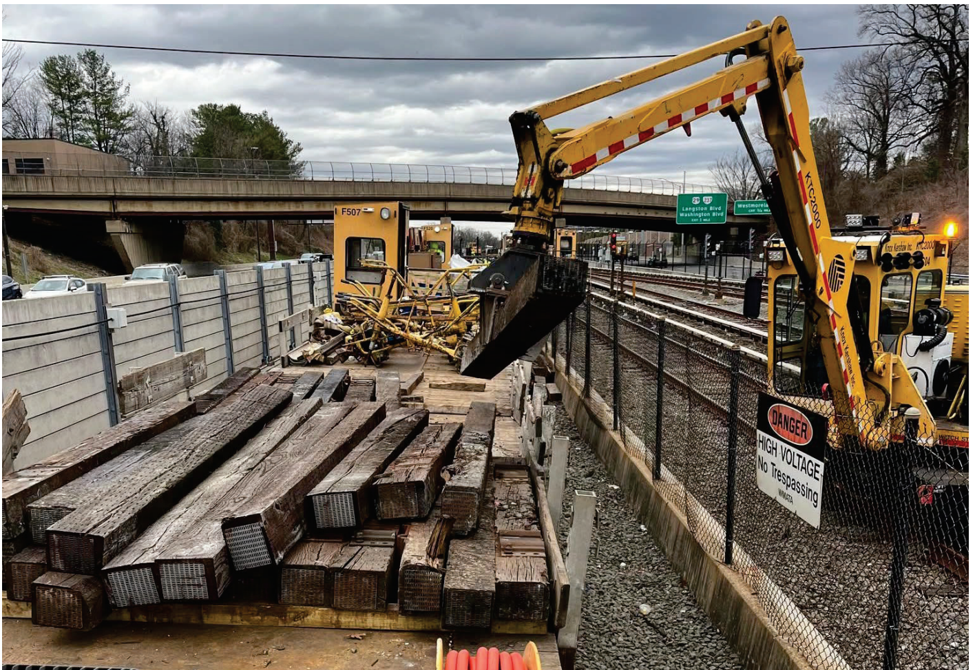
Pictured: Metro Rail preventive track maintenance
