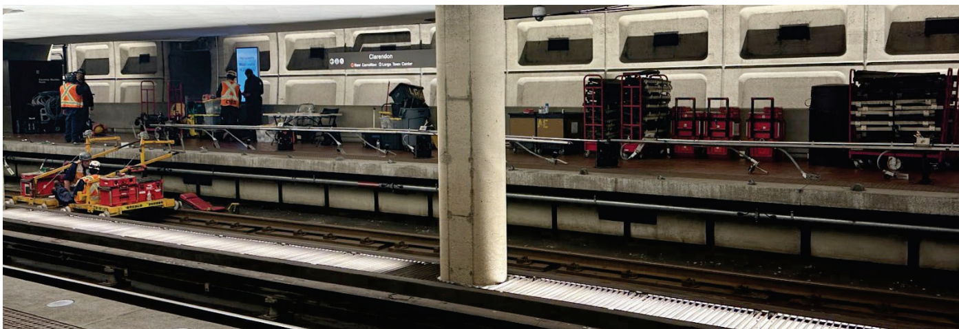
Pictured: Workers replace electrical infrastructure along a Metro station's platform edge
