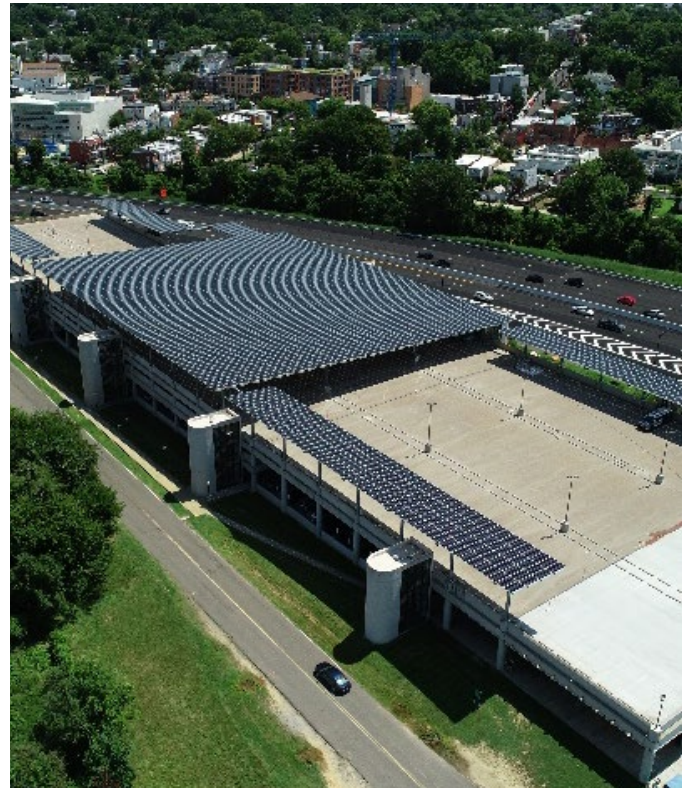
Solar Carports at Anacostia Station Garage (Aug 2022)
