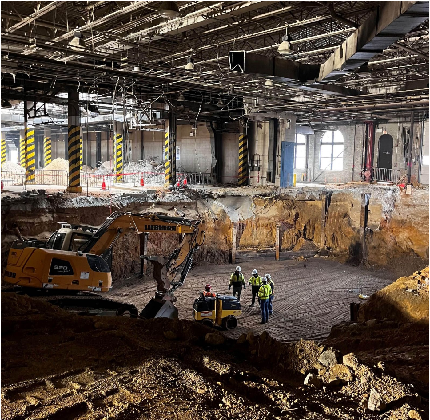
Northern Bus Garage construction
