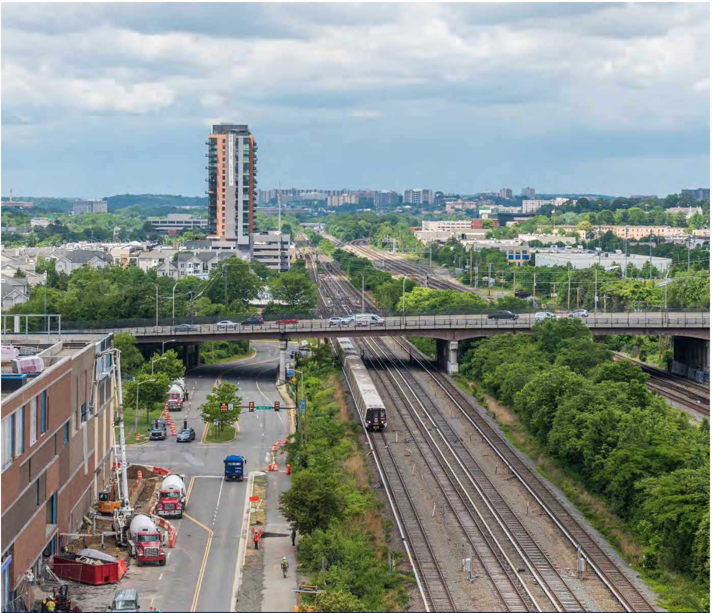
Construction for new Metro office and larger redevelopment near Eisenhower Ave Station
