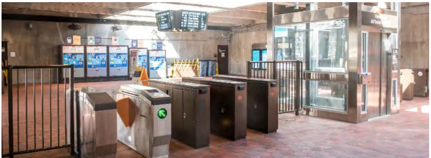
New faregate at Dunn Loring Station
